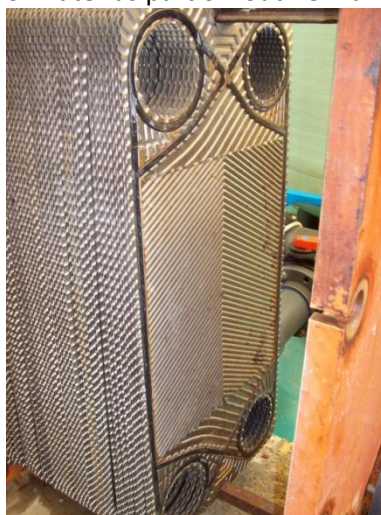
Figure 7: A heat exchanger protected against limescale by HydroFLOW. Instead of twice-yearly acid washes, the exchanger is hosed down once a year as part of routine maintenance.
