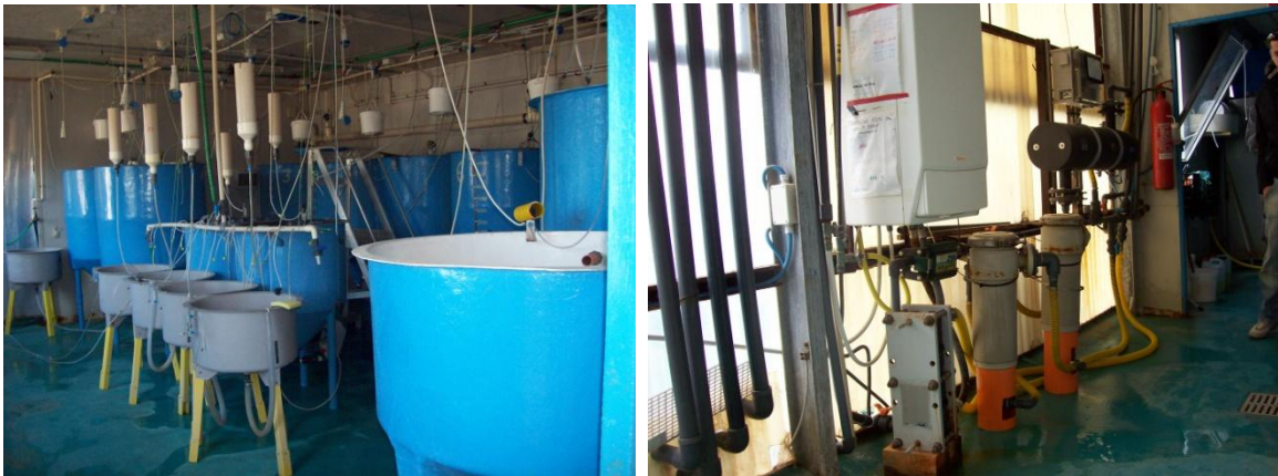
Figure 5: In these tanks (Right), new-born fish are placed to begin their growth. The HydroFLOW unit (right) protects the fish against bacteria, and also protects the heat exchanger against limescale.
